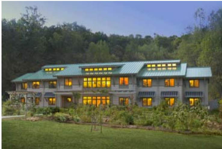
EcoDorm Warren Wilson College – LEED EB Platinum Samsel Architects, P.A
