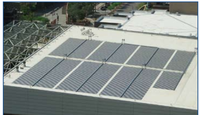
Phoenix West Convention Center Photovoltaic Roof System Installation
