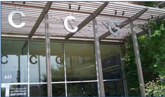
Chicago Center for Green Technology (CCGT) Renovation
