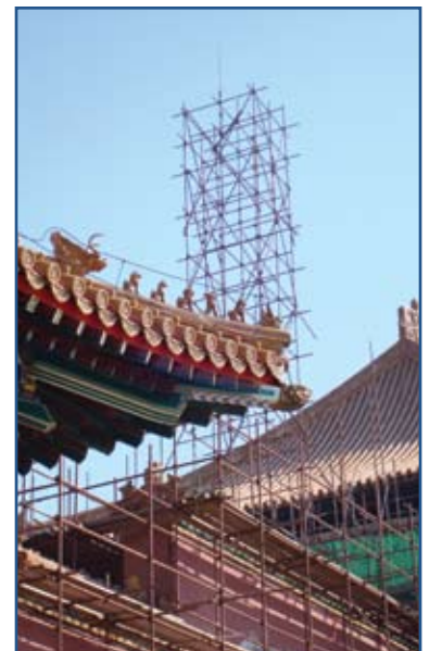
Forbidden City in Beijing under renovation.
