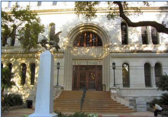
City Hall, San Antonio, TX
