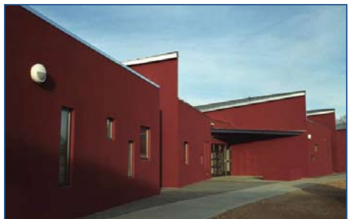
Agua Fria Elementary School Repairs and Upgrades
